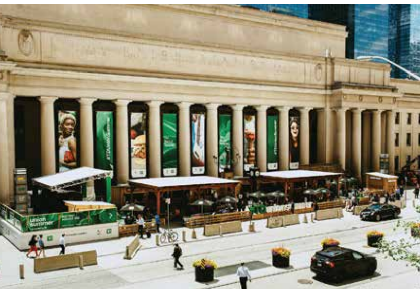
ABOVE: Toronto's Union Station, undergoing a multi-year renovation, partnered with A&C to help bring its vision, new brand, and programming to life. The agency developed a strategy that ensured sponsors would create value-adds and enhance the overall experience, ultimately securing TD Bank.
